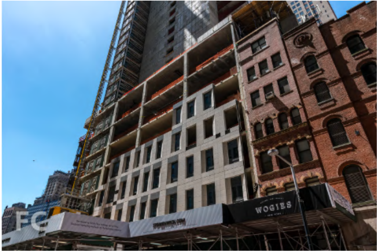
Looking up at the east facade.
