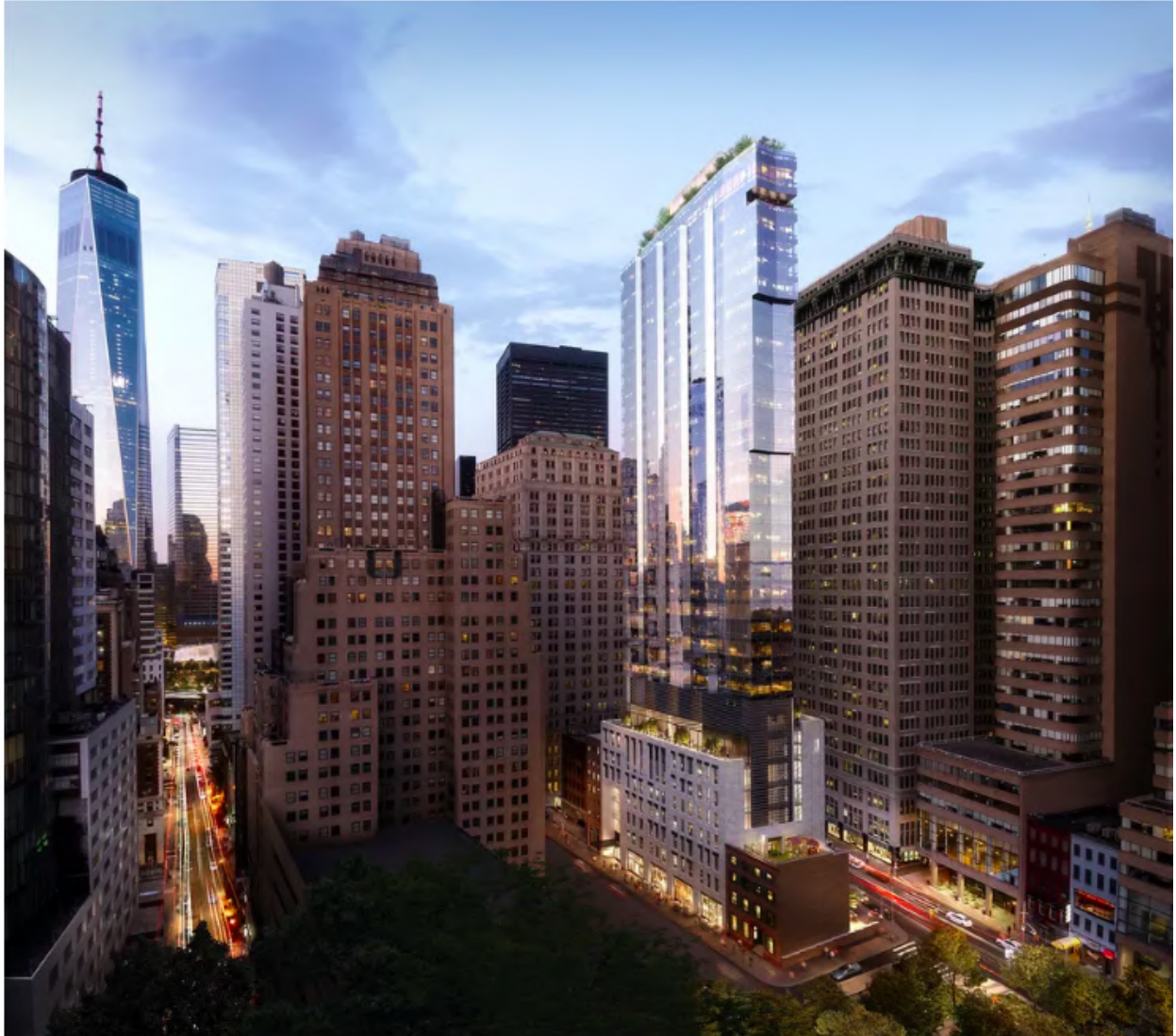
The building was approved by the Landmarks Commission in 2016.
