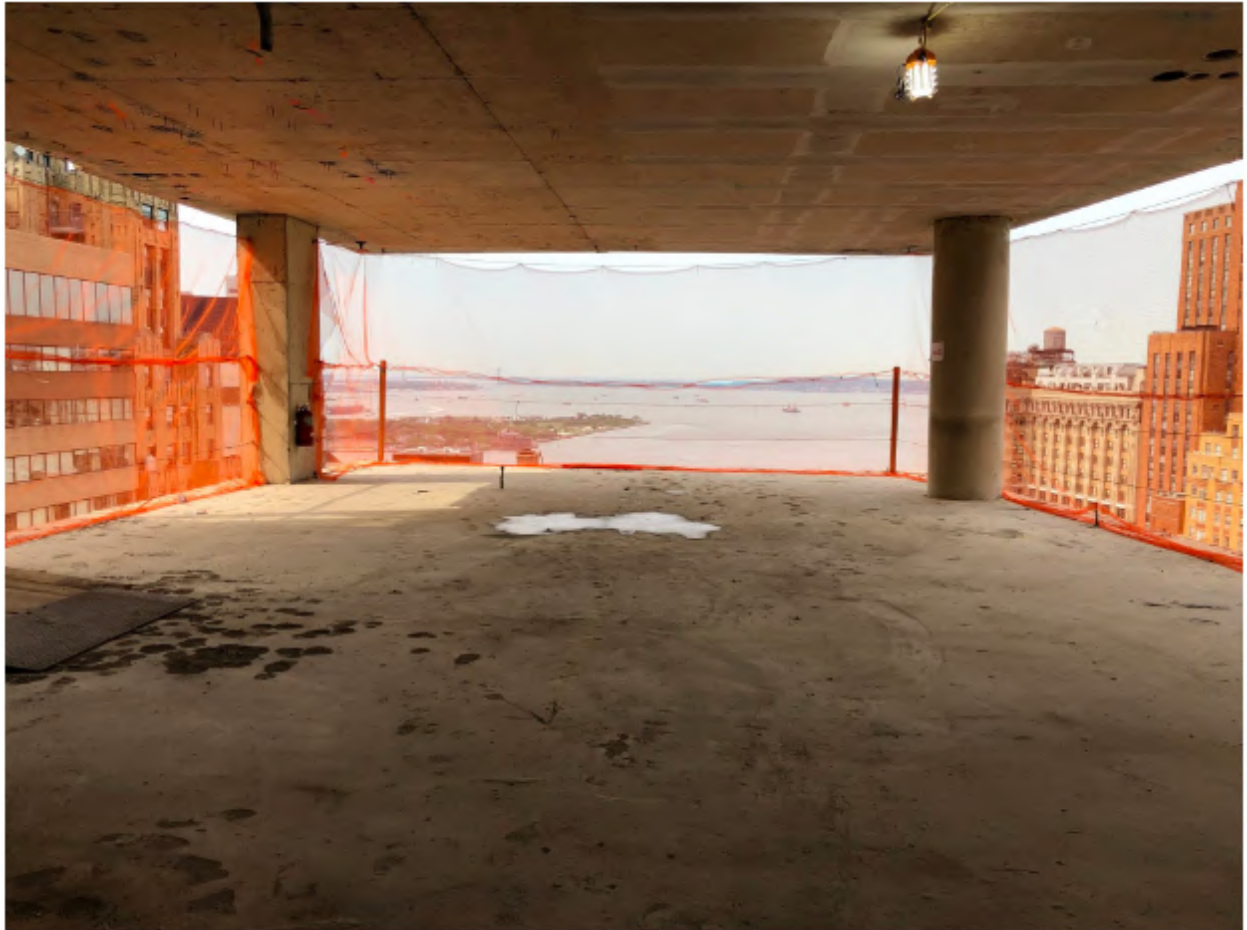
One of the upper floors with perfect views of the harbor. Photo by Michael Young
