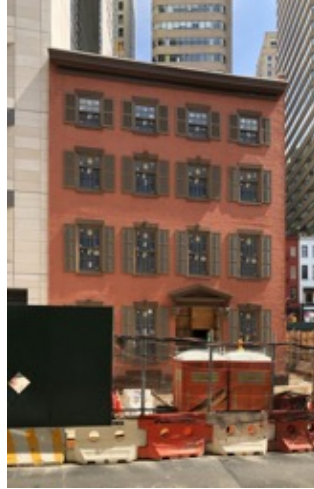
The western elevation of the Robert and Anne Dickey House. Photo by Michael Young
