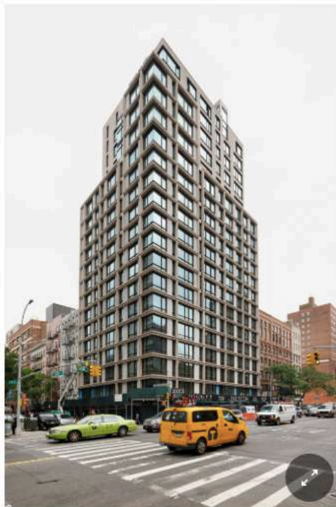
The luxury condominium at 200 East 21st Street in Gramercy is the latest green project from Alfa Development. The 20-story, 67-unit building has high-performance glass to reduce solar gain, landscaped "green roof" areas and motion-controlled LED lights in the common spaces. Stefano Ukmar for The New York Times
