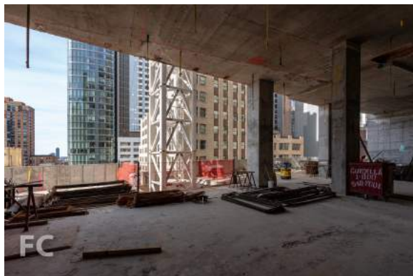
Tower crane support at a lower tower floor.
