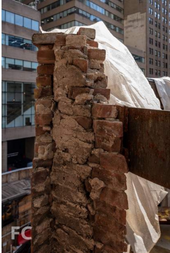
Closeup of the facade of the Dickey House.
