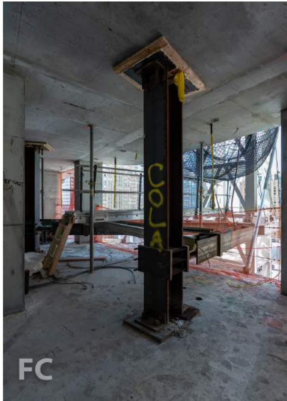
Tower crane support at a lower tower floor.
